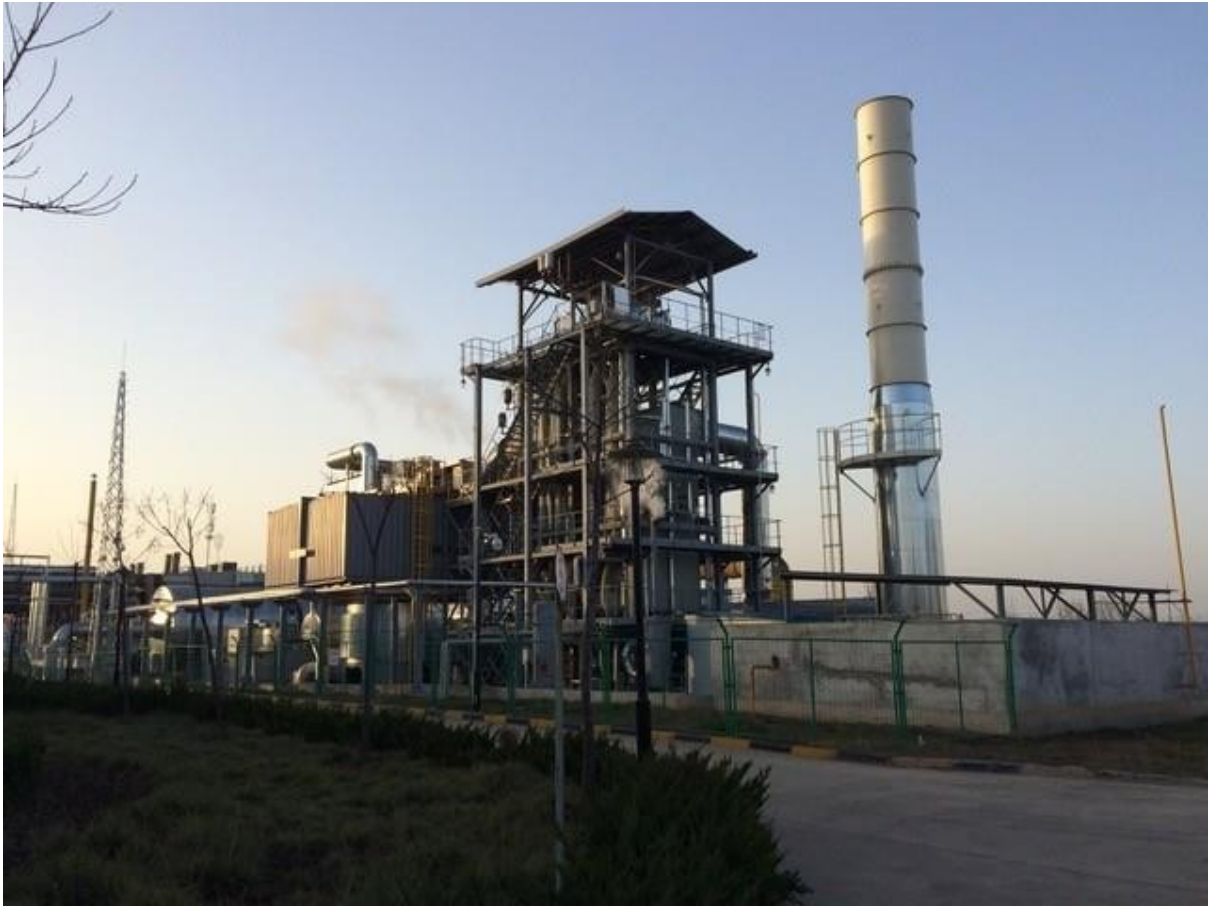
Dafosi Coalmine, Binchang, China
