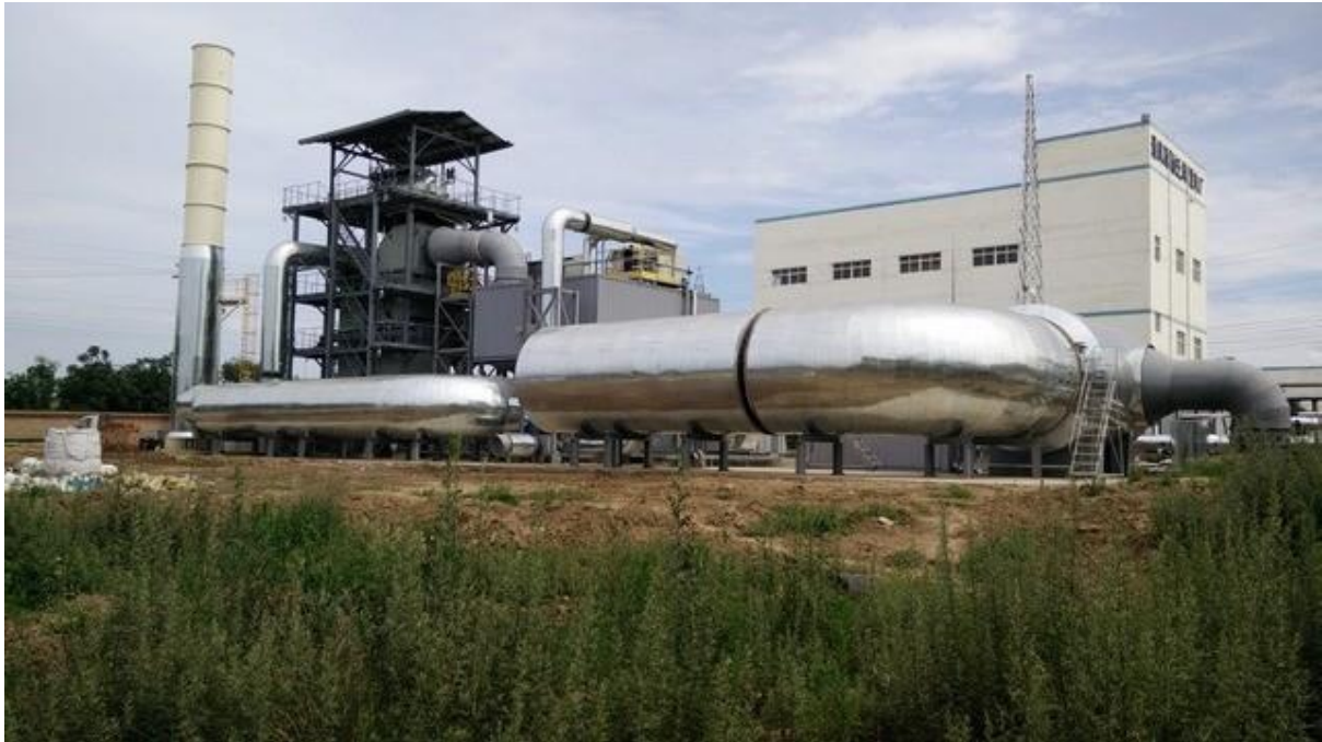
Dafosi Coal mine, Xianyang City, Shaanxi Province, China
